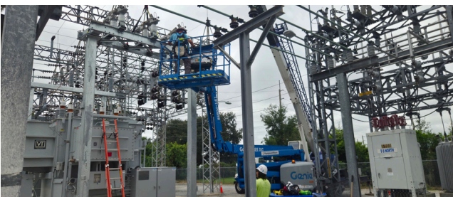
INDUSTRIAL ELECTRICAL CONSTRUCTION
