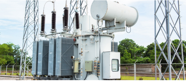
TRANSFORMER TESTING, REMEDICATION AND REPLACEMENT
