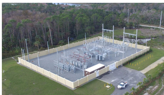
ELECTRIC SUBSTATION CONSTRUCTION
